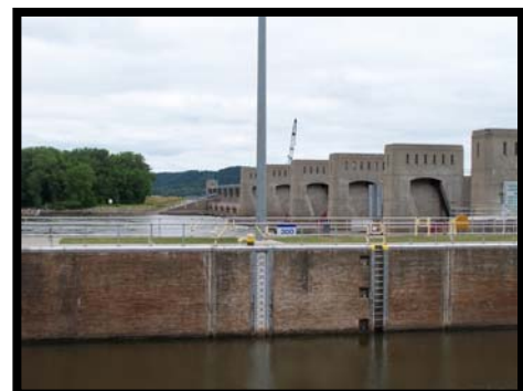
Mississippi River Lock and Dam 9
